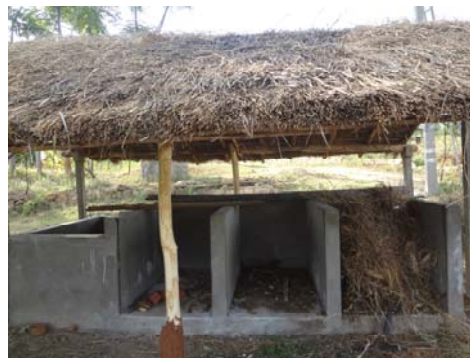
Hot compost pit under the shed
