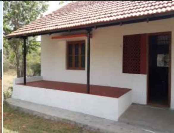
Dormitory in 2019 after renovation
