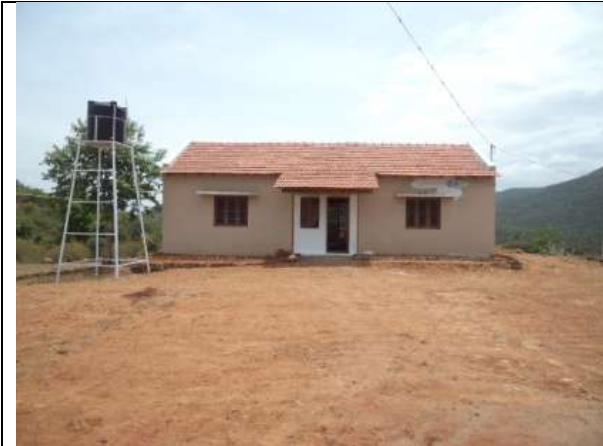
Dormitory in 2012 before renovation
